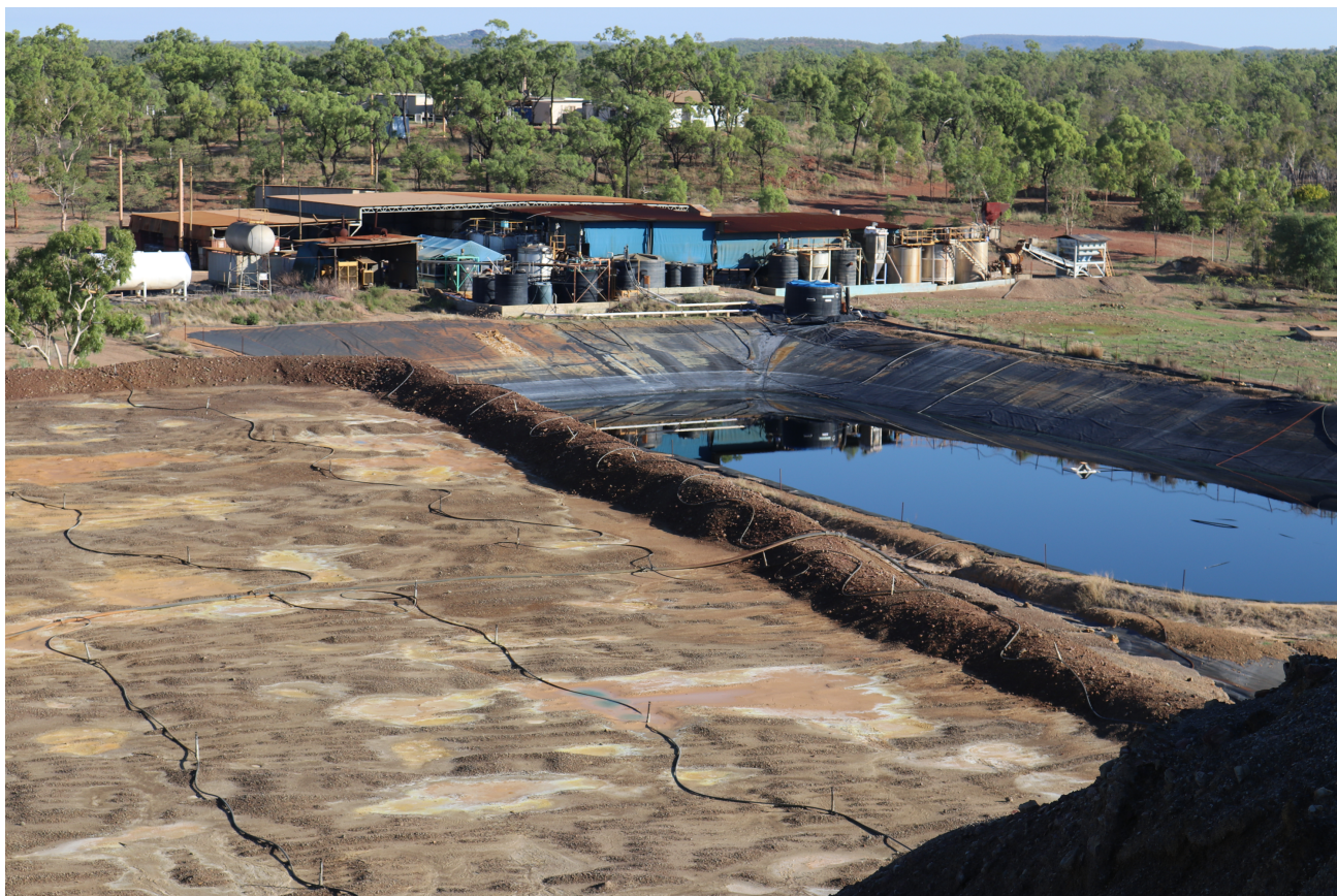
Above: Aerial view of the Tartana Plant
