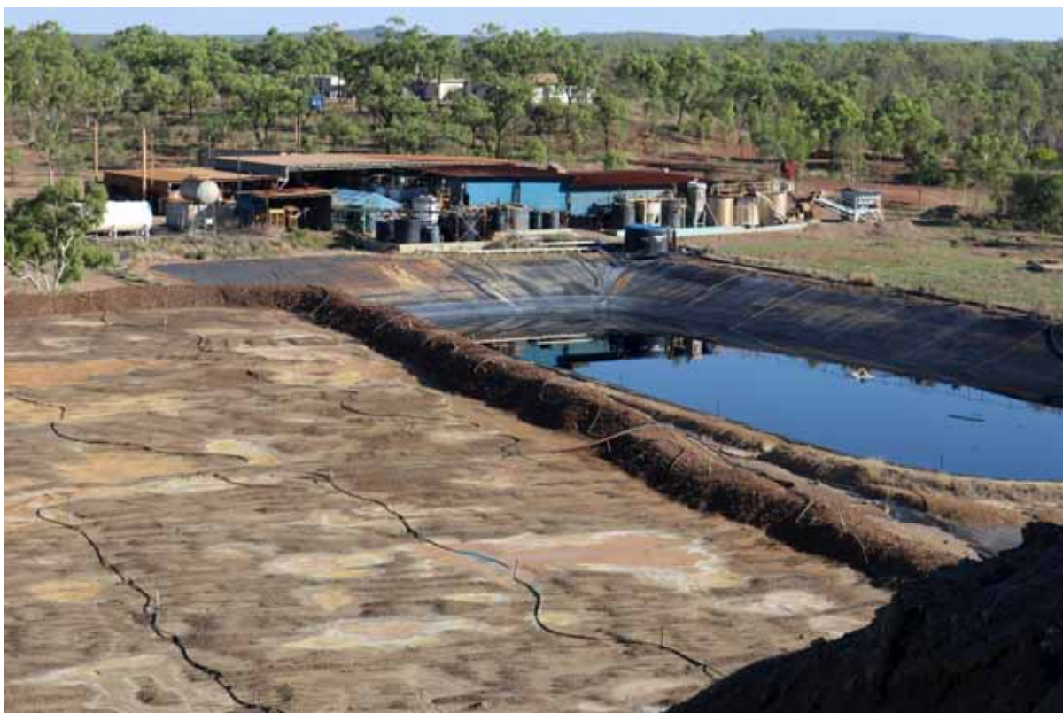
Figure 5– Heap leach pads and Solvent Extraction plant. Accommodation village in the background (9 December 2017)
