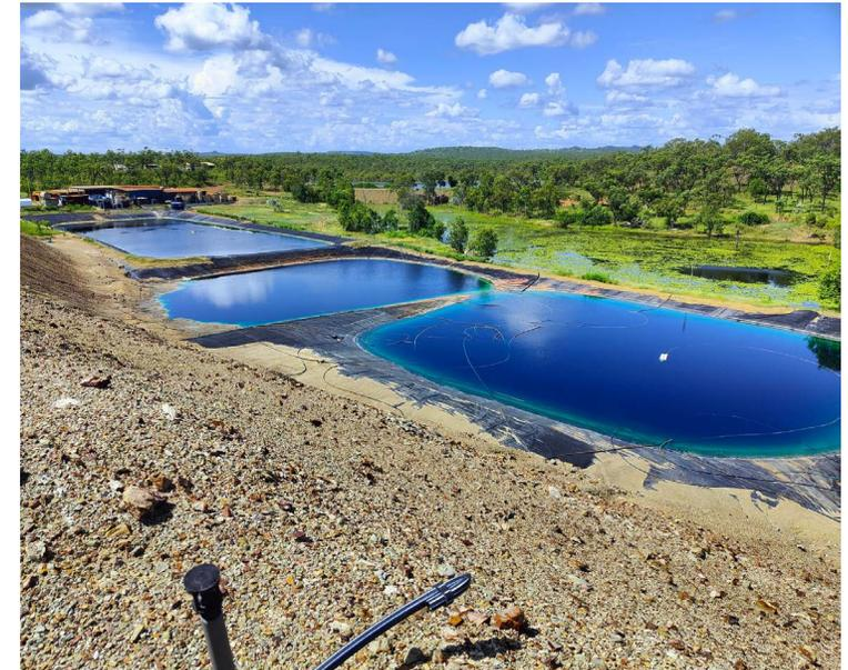
The heap leach – solvent extraction – crystallisation circuit is similar to a heap leach solvent extraction – electrowinning plant (e.g. Nifty Copper Mine (ASX:CYM), Capricorn Copper Mine (ASX:29M)) except we produce copper sulphate instead of cathode copper. Copper Sulphate sells at a premium to the LME copper price but generally has lower operating and capital costs.
