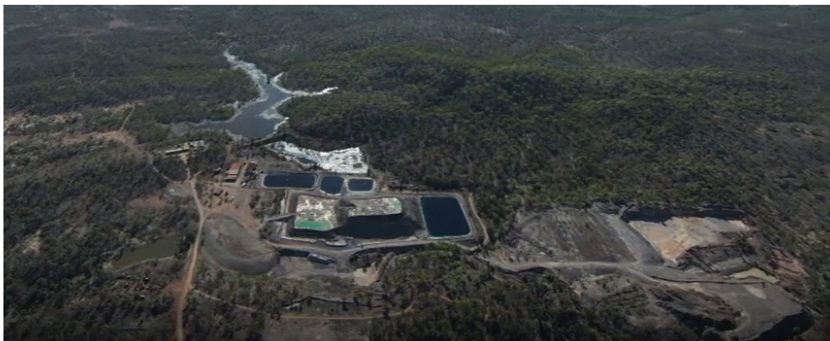
Figure 2. Aerial view of the Tartana mine site in August 2022.
