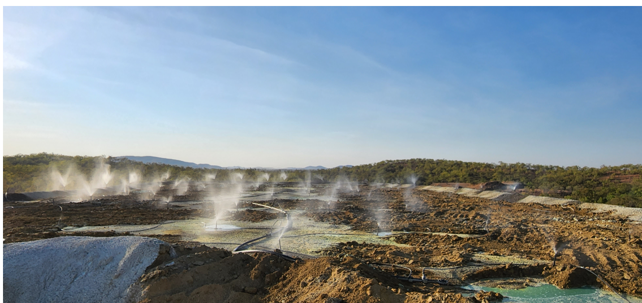
Figure 2. Turning of the top and bottom heap leaches.
