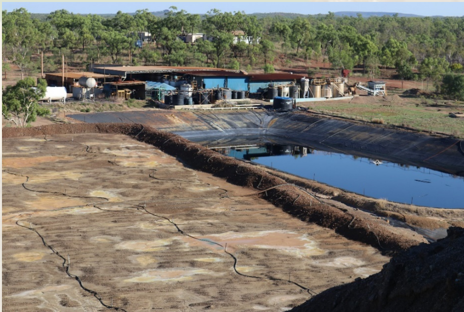
Heap leach pads with plant and accommodation camp in the background (above). Copper sulphate in feeder and liquor tanks (right)
